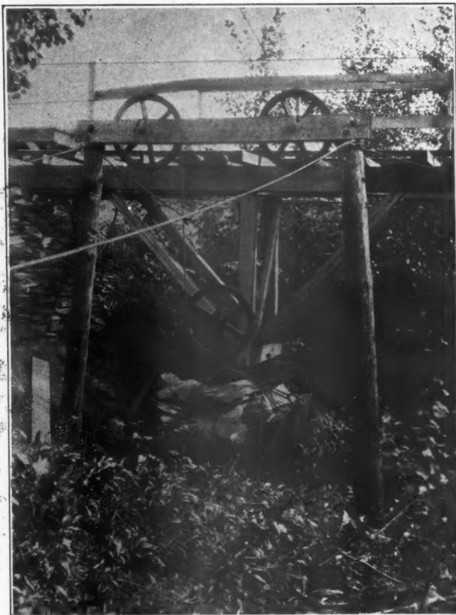
Counterbalance for Wire Rope Controlling Car to Slate Mill
